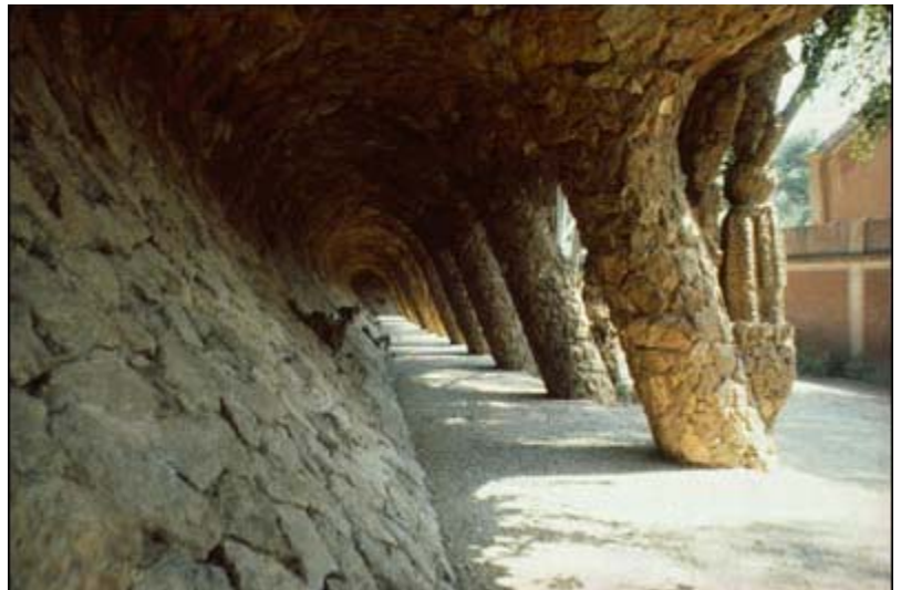
A covered walkway in the Parc Güell shows off one of Gaudí's signatures: the parabolic arch.
