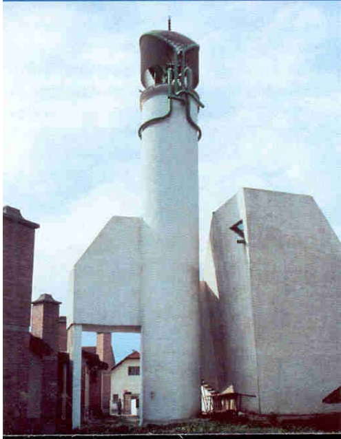
Contemporary architects reinterpret traditional forms: Sherefudin's White Mosque in Visoko, Bosnia-Herzegovina won an Aga Khan Award in 1983. It is now destroyed.
