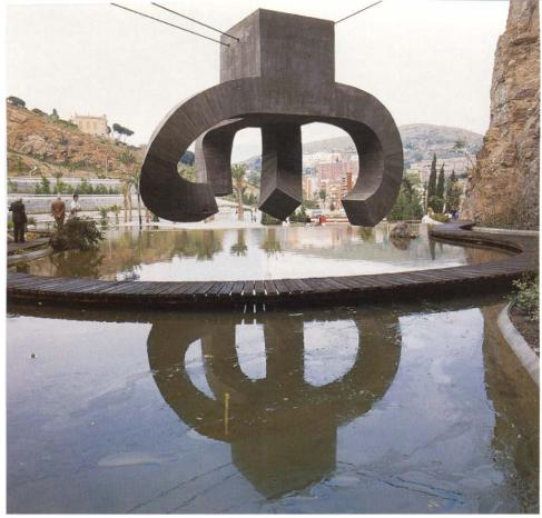
*Eulogy* to Water (left) was commissioned in 1987 for a city park in Barcelona. The precast concrete structure is suspended on steel cables from surrounding cliffs.
